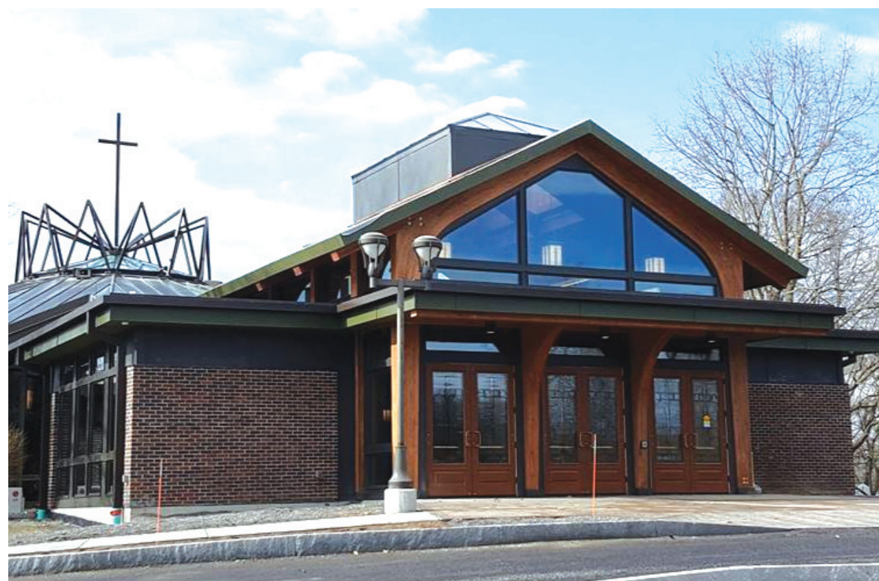
The current I.C. Church. Fourteenth pastor, Rev. Thomas Ryan, oversaw a major renovation which included expanding the main entrance with this large gathering vestibule.
